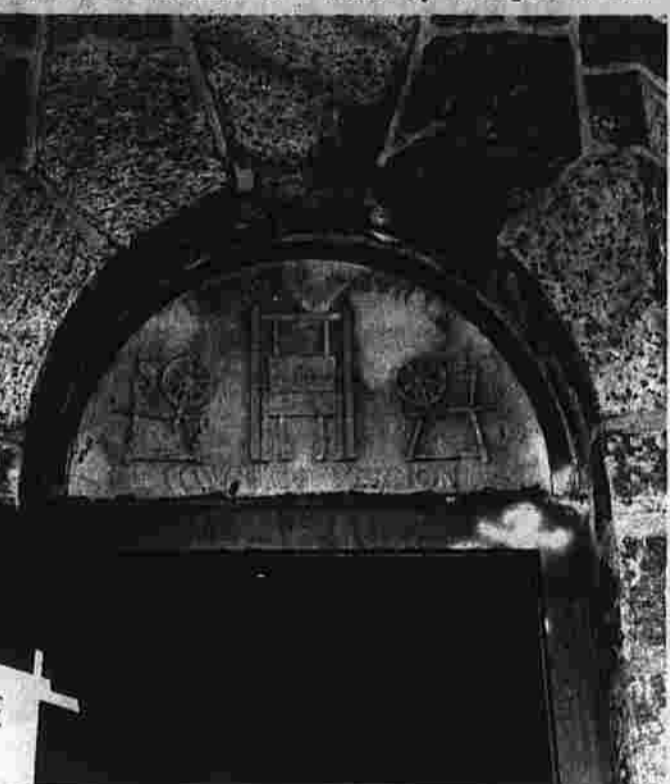
(Photo by Barbara Richmond) Doorway at Fox Hill Tower, Rockville.
